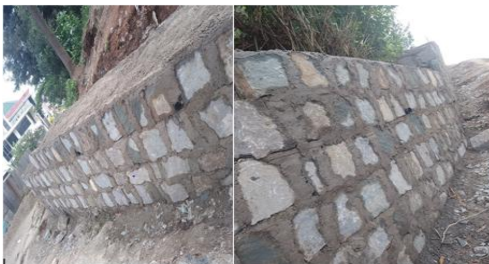
Figure 11 Flood Walls Found in Addis Ketema Sub City.
