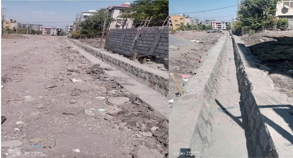
Figure 9 Inner Road Drainage Constructions by Community Participation in Akakai Sub City
