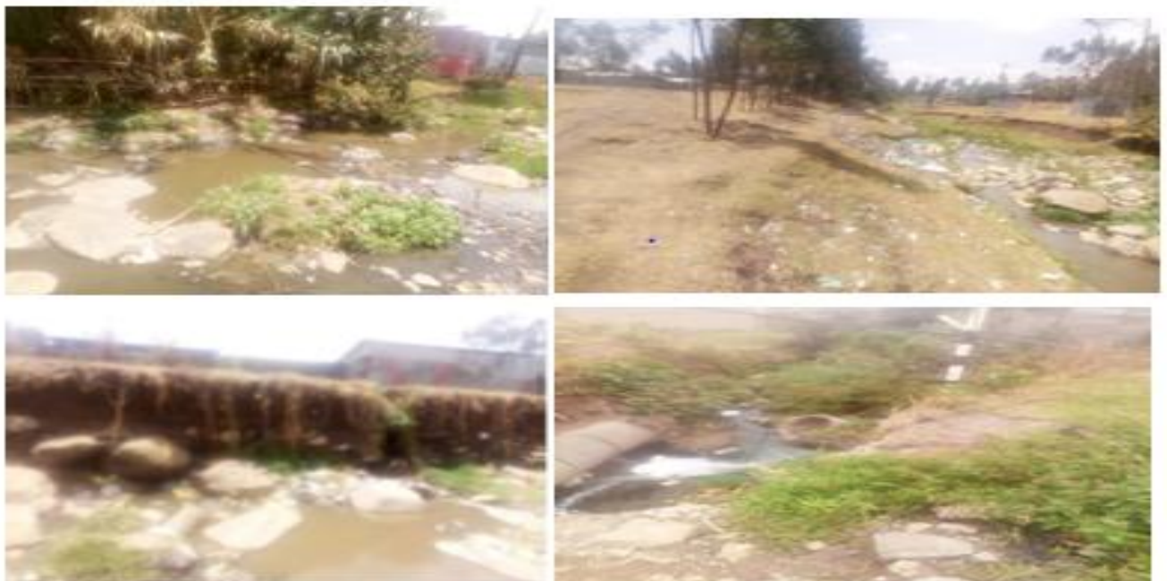
Figure 6. Flood Prone Areas in the city. Source: AAFDRC, 2024
