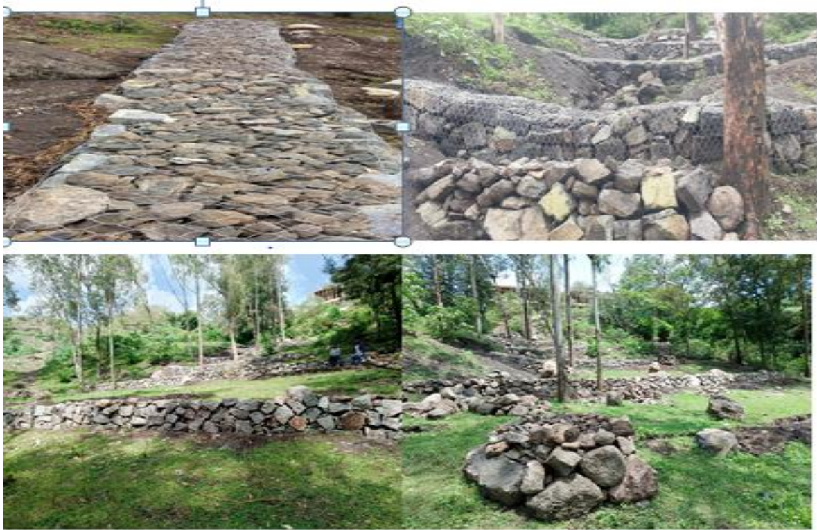
Figure 12 Terracing Works in Akaki Sub City.
