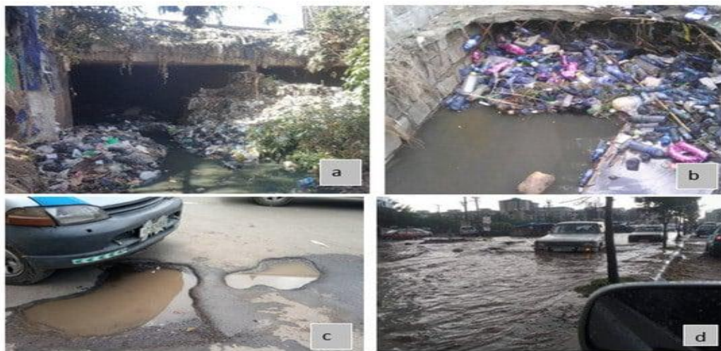
Figure 14 Solid Waste Blocked, Drainage System in Addis Ababa City
