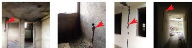
Fig. 4.8 Chiseling rework after masonry work is over
