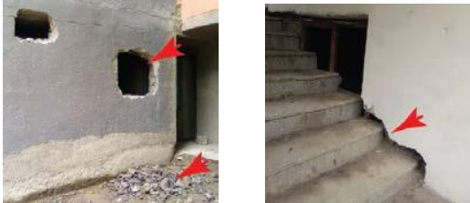
Fig 4.7 Rework wastage observed in sample sites
