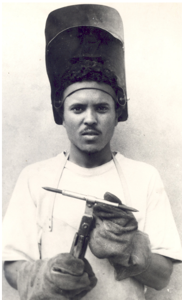
Fig. 3. Arc welding operator inserting the special carbon electrode into the electrode holder of an electric arc welder.
